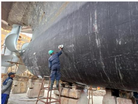
Figure 9: Installation of new anodes
