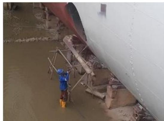
Figure 10: Protective recoating of ship's hull
