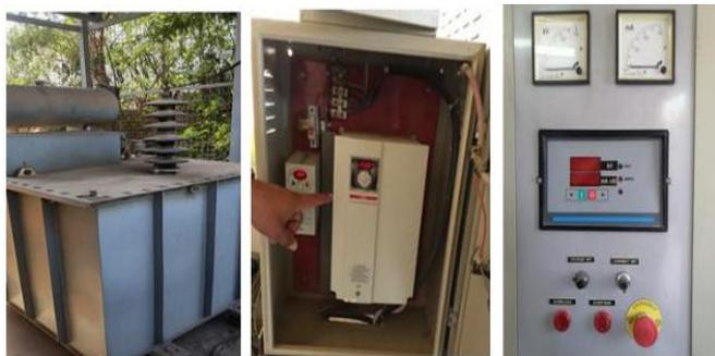
Figure 2: (a) DC Power Supply for ESP, (b) Fan Variable Speed Driver, (c) The main control panel of ESP
