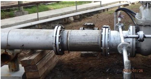
Figure 1: Flexible Joint at the piping system
