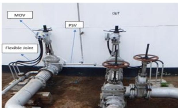
Figure 3: Location of MOV and PSV in relation to the flexible joint of the storage tank
